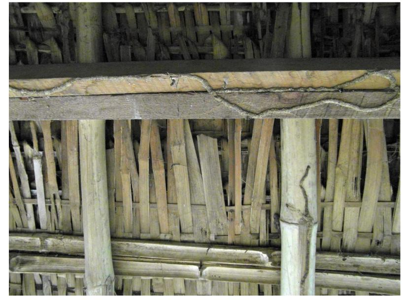
The truss is made of beams and bamboo.
